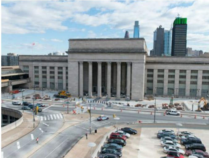
The re-designed west entrance of 30th Street Station. (Credit: Amtrak)
